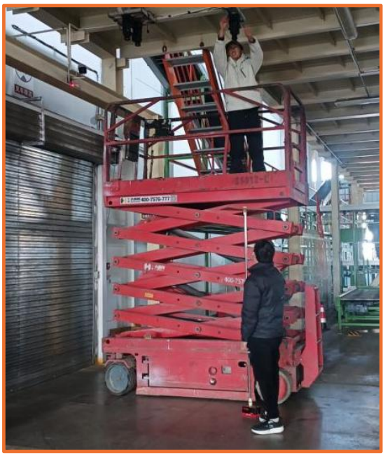
现场安装投影灯
